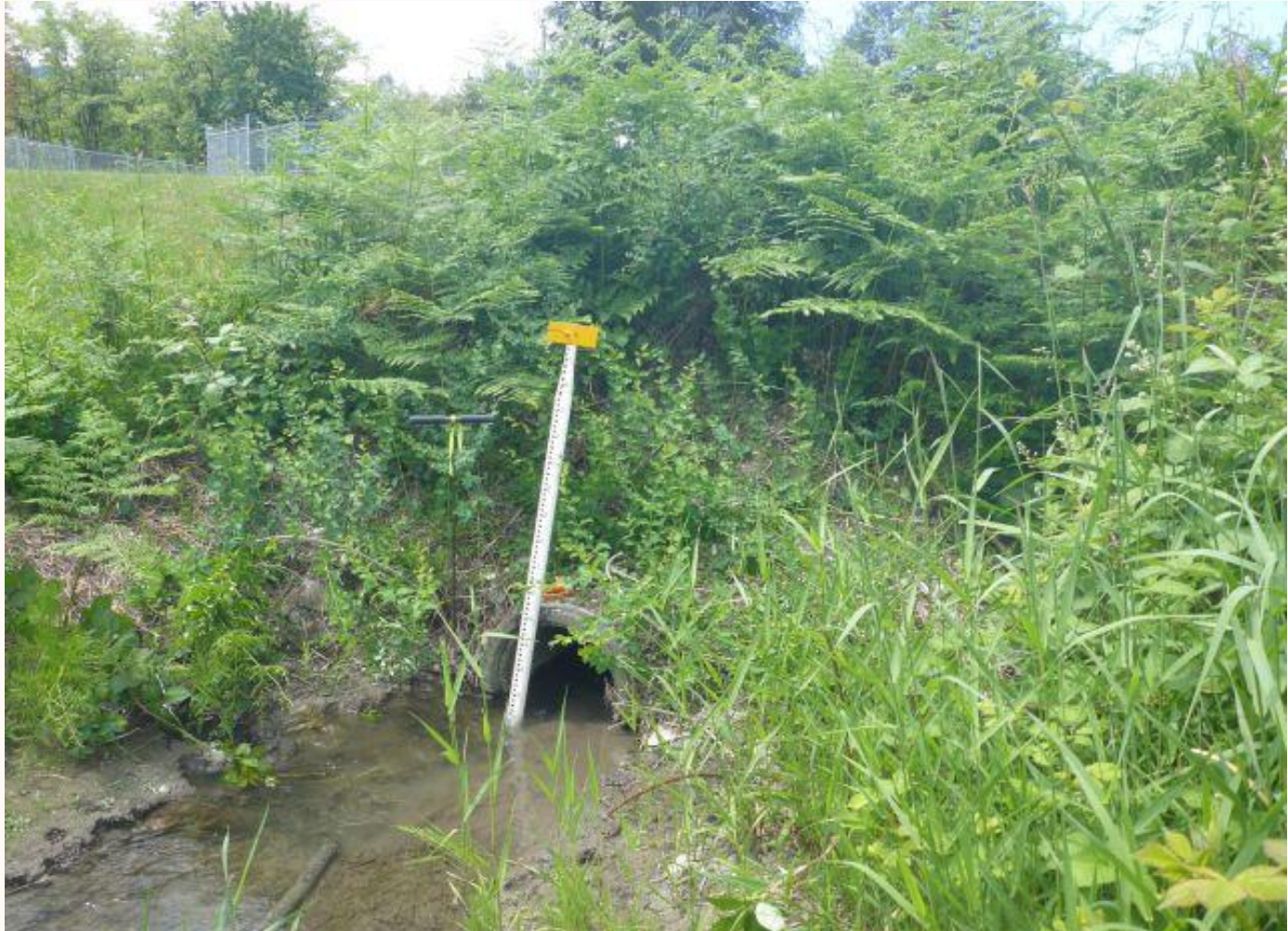
Inlet to piped portion of Lorenzan Creek under road shop.
